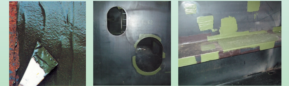
Thick film of Nu-FORTE Barrier easily to cover the gap after surface preparation
