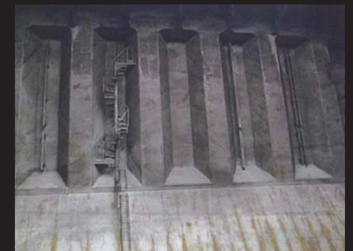
Ballast tank and hold (double use) in 90,000 DWT coal carrying vessel
